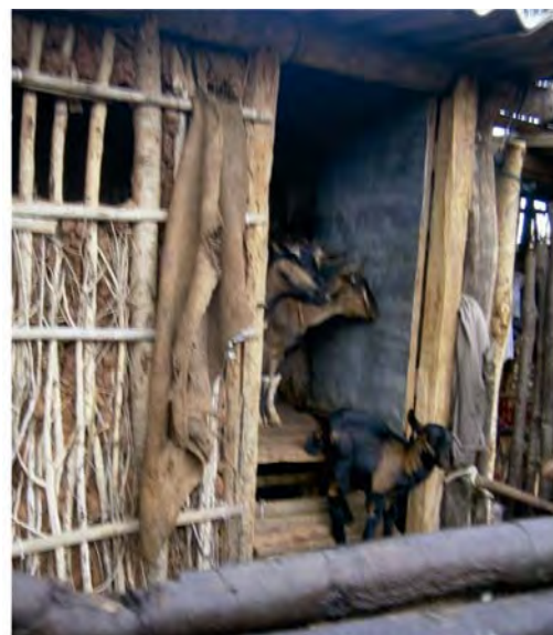
Goat shed constructed on a raised platform
