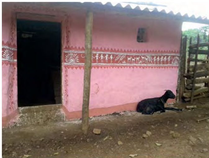
A recently constructed goat shed at Palami village in the Patakhonda cluster in the Sudra gram ganchayat
